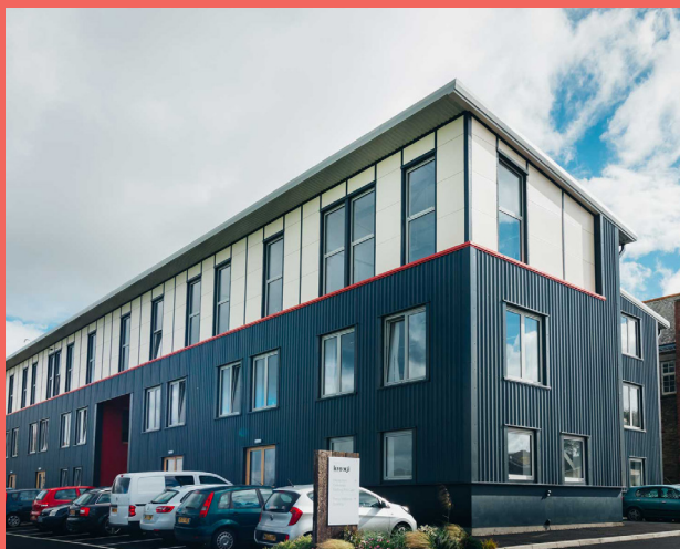
The ERDF-supported Percy Williams Building at Krowji © Krowji, Kirstin Prisk Photography
